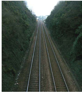
Figure 1 The receiver's view off all but the highest-elevation satellites is severely restricted by deep cuttings
