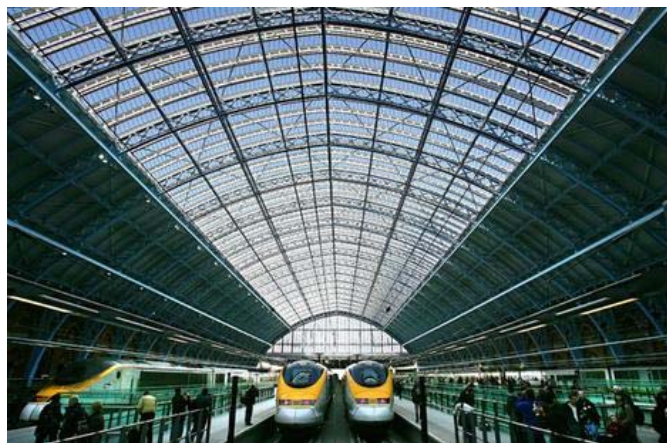
Figure 2 Overall roofs such as this at London's St. Pancras station not only attenuate satellite signals, but the complex metallic frames that form the structure can also cause multipath problems
